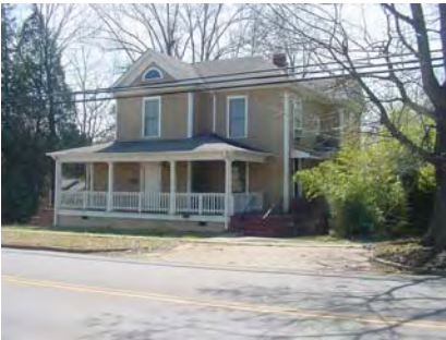
401-A-D Charlotte Ave Rents: $385 - $495 Deposits Vary 1 BR and 2 BR units Porch, Two decks
